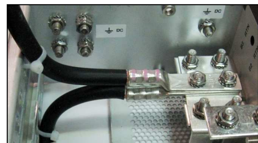
Fig. 10b – Return Cable Strain Relief
